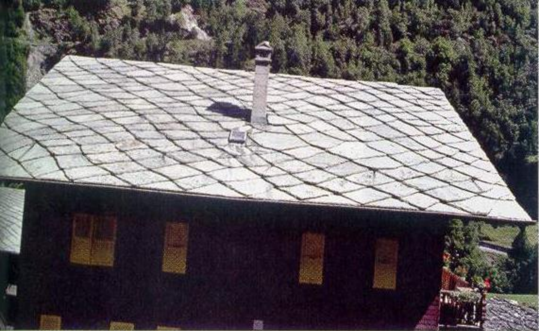
Figure 7.7 Slate used for roofing material on a house in Switzerland. (Photo by E. J. Tarbuck)
