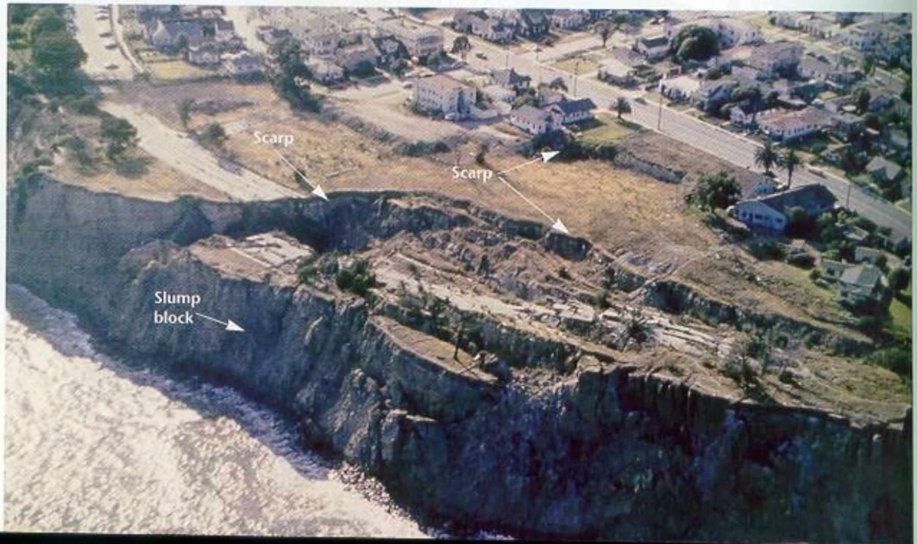
Figure 9.9 Slump at Point Fermin, California. Slump is often triggered when slopes become oversteepened by erosional processes such as wave action. (Photo by John S. Shelton)
