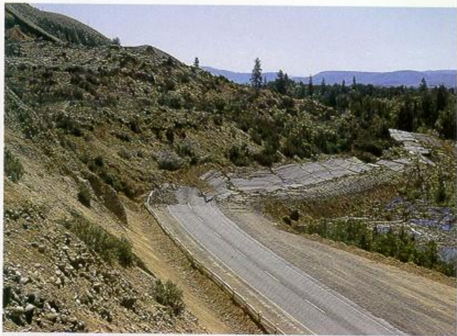
FIGURE 8.4 A large slump in a high gravel terrace beside the Yakima River in central Washington has broken up a major highway and displaced it more than 100 m laterally into the river channel
