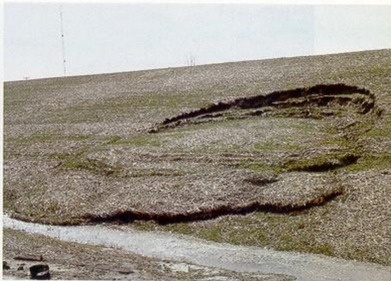
Figure 9.14 This small, tongue-shaped earthflow occurred on a newly formed slope along a recently constructed highway. It formed in clay-rich material following a period of heavy rain. Notice the small slump at the head of the earthflow. (Photo by E.J. Tarbuck)
